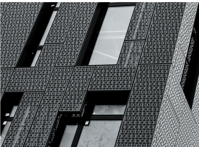
EOLAS Building, Maynooth University, Co. Kildare
